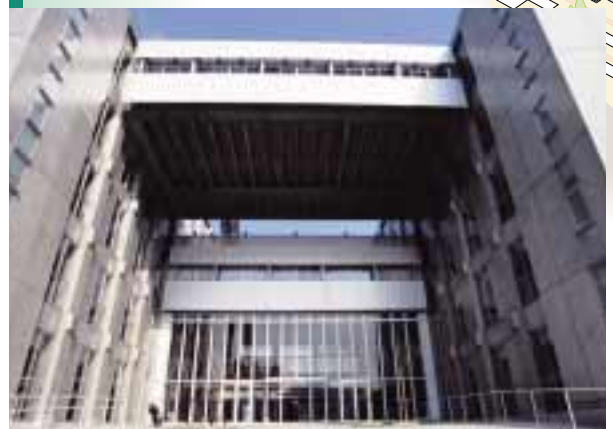
Uji Research Building 11,199m 2 (Bioinformatics Center)
