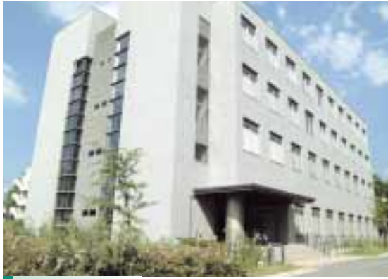
Joint Research Laboratory Building 3,777m 2
