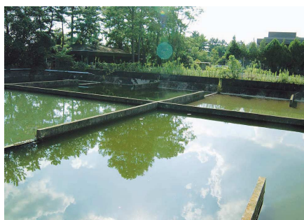
Drainage Monitor Center of Uji Campus
