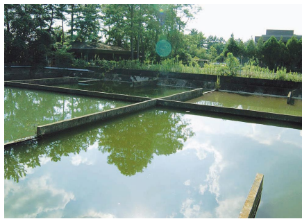
Drainage Monitor Center of Uji Campus
