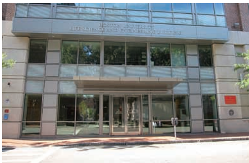
A Bioinformatics Program's building (Life Science and Engineering Building, Boston University)
