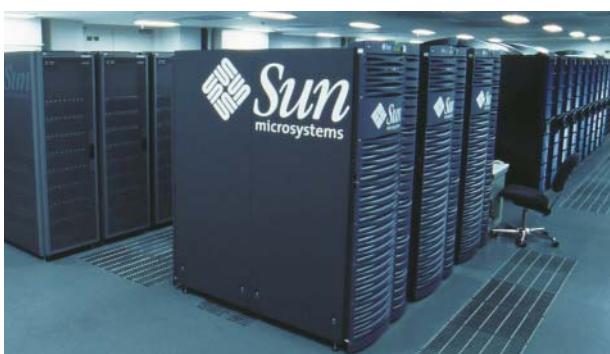
GenomeNet Server on the first floor
